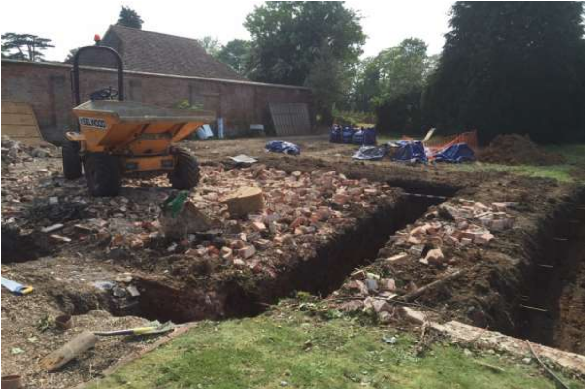
Plate 2. General view of site showing demolished garage and new foundation trenches (looking south- west)
