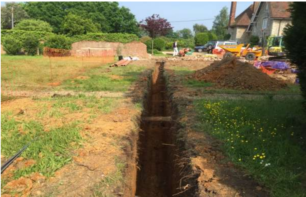
Plate 5. View of the garden wall foundations (looking east)
