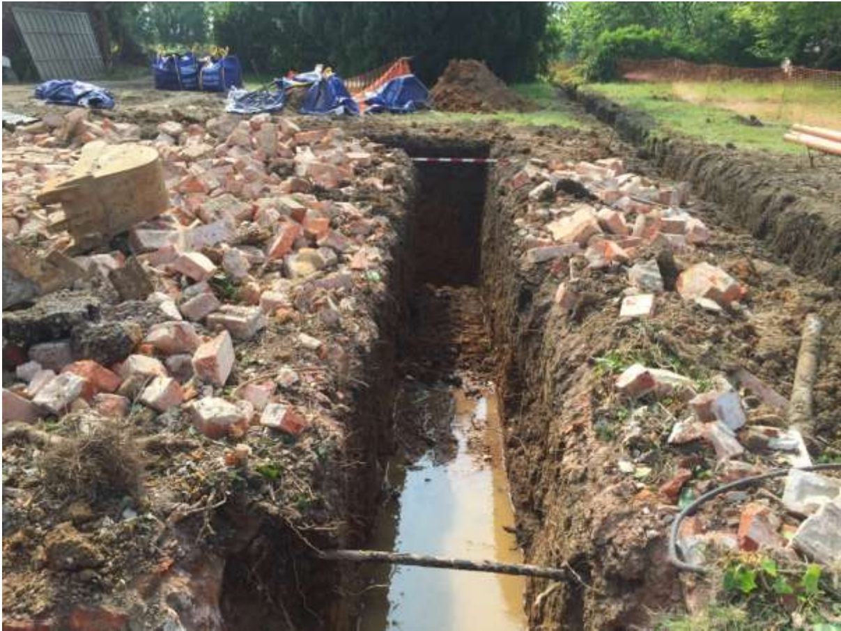
Plate 4. View of the garage foundation trenches (looking west)
