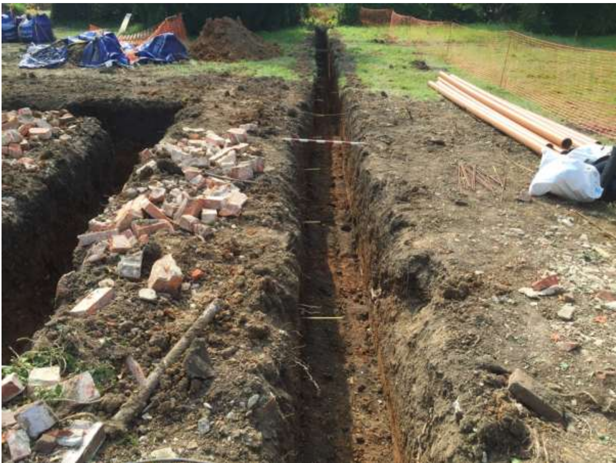
Plate 7. View of garden wall foundation trenches (looking west)
