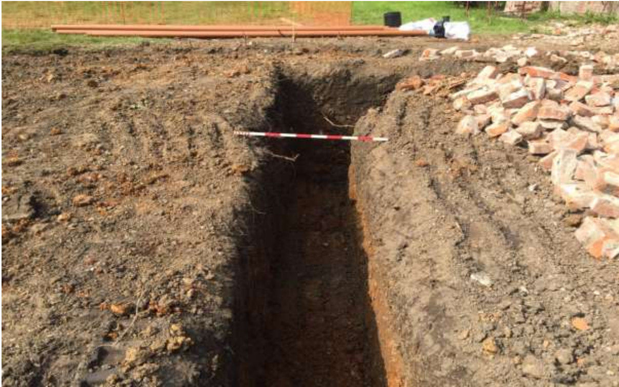
Plate 6. Cutting of garage foundation trenches on south side (looking west)
