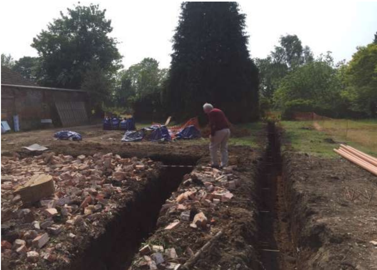
Plate 3. View of the new garage and garden wall foundation trenches
